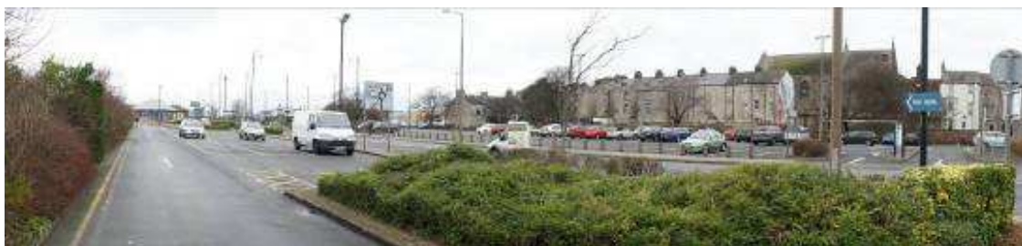
Telephone Exchange Car Park and Morecambe Station car park
